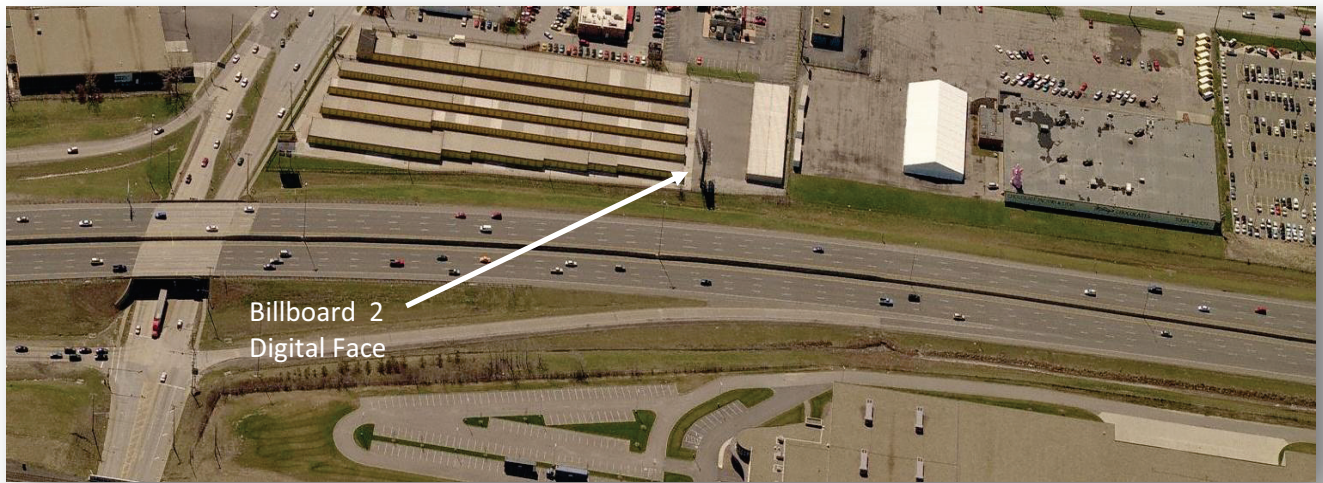
Figure 10. Oblique Aerial of Digital Billboard 2 on I-480
